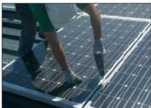
Serreur entre PV Clamp between PV modules
