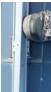
Clipper au pied le rail Clip the rail by foot
